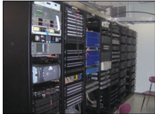
The heart of the tech center is the blue dual-framed SAS 32KD router cabinets. In the far racks you can see some of the many BE Audiovault workstations that are extended to studios and offices by the Avocet KVM system.
